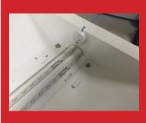
**LED Light** is Visible. Sensor is Not **Pointed Toward** the Floor.
