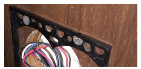
Photo 10: Example of improper screw used for surface mount installations.
