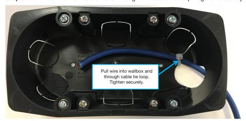
Photo 9: Visual instructions for step 3 of the cable retention assembly.
