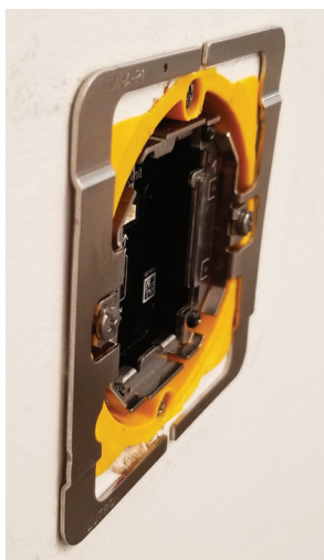
CORRECT Adapter flat against wall.
