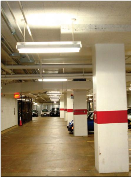
By replacing this legacy lighting system with new fixtures, dimming ballasts and occupancy sensors, one State Department building garage saved more than 400,000-KWh, or about \$64,000 in electricity costs, annually—an estimated 83 percent energy savings from the baseline.
